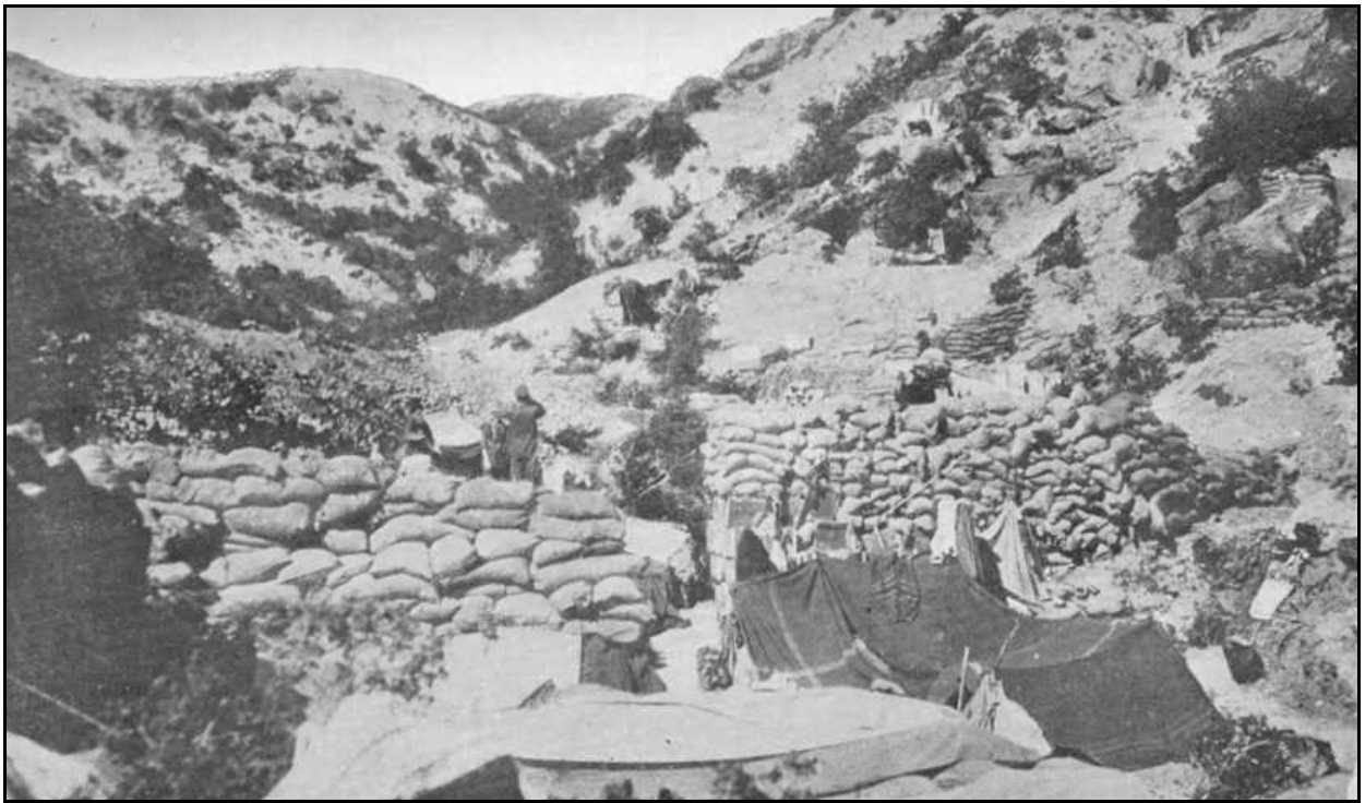
A scene in Shrapnel Valley (Monash Gully) as the Turkish snipers at the head of Monash Gully could enfilade stretches of the road; sandbag traverses were built at the most dangerous points
